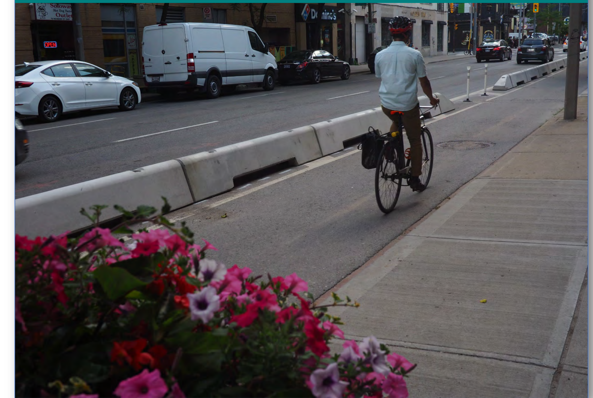
Example of concrete low-wall barriers
