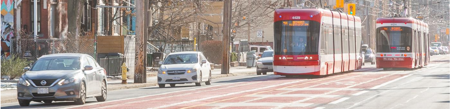
Red streetcar priority lanes installed in 2025 on Bathurst Street near Carr Street, looking south.
