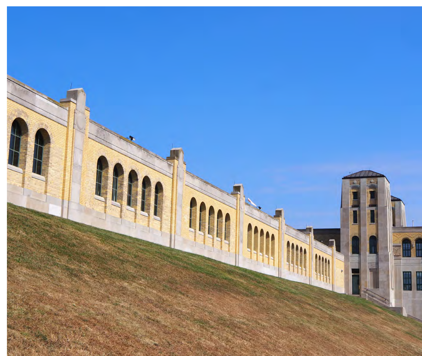
R.C. Harris Water Treatment Plant
