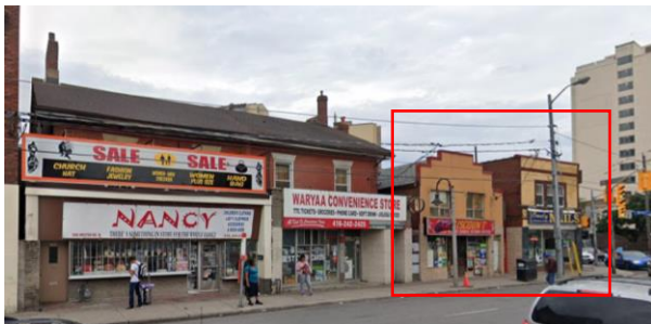
Figure 28: Weston Road south of Lawrence Avenue West, 2019. The gable roof is visible behind the brick façade on the property at 1894 Weston Road (Google Streetview)
