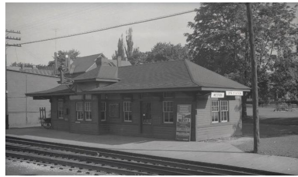
Figure 17: CPR Station near Rosemount Avenue and John Street, 1953 (Toronto Public Library).
