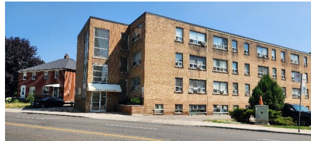
Figure 42: The Westlyte Apartment building at 2275 Weston Rd was the first constructed in this area (Heritage Planning, 2025).
