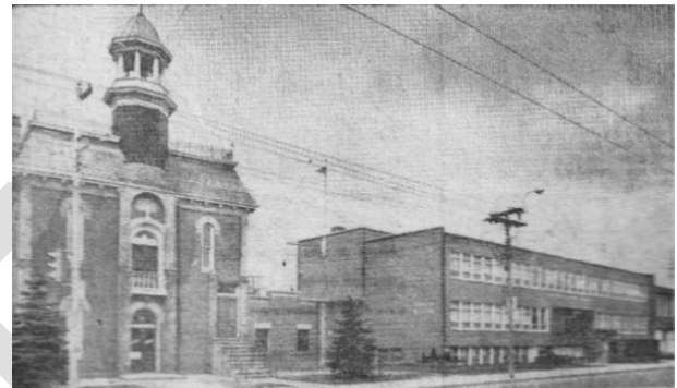
Figure 10: Weston’s old Town Hall (left) and new Municipal Building (right) prior to the demolition of the old Town Hall in 1964 (Weston Historical Society)
