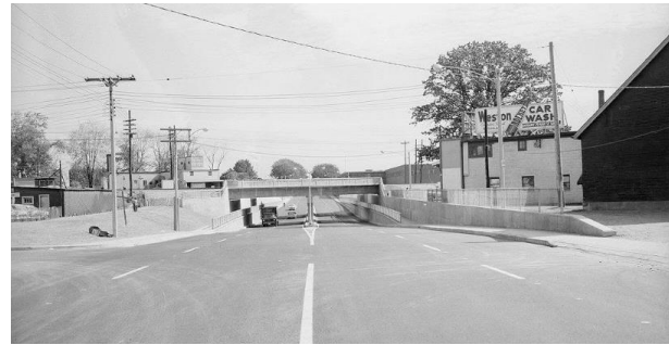
Figure 15: Lawrence Avenue West with newly constructed underpass, looking east from Weston Road, 1960 (City of Toronto Archives).
