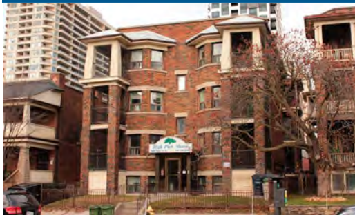
Showing principal (south) façade, looking northwest (Heritage Planning, 2023).
