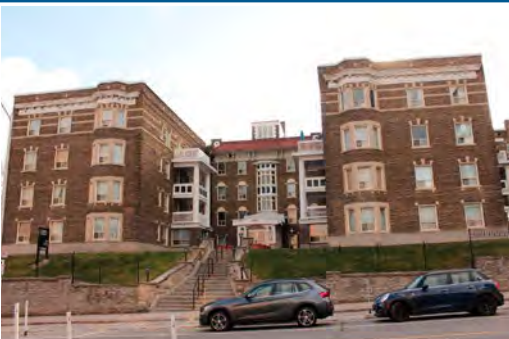
Showing principal (north) façade, looking south (Heritage Planning, 2023).
