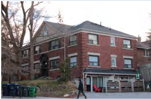
Showing principal (north) façade and west façade, looking southeast (Heritage Planning, 2023).
