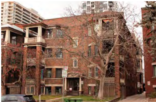
Showing principal (south) façade, looking northwest (Heritage Planning, 2023).
