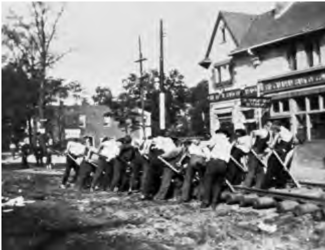
Laying Bloor Streetcar line west of Runnymede Road, 1917. (Swansea Historical Society 2018)
