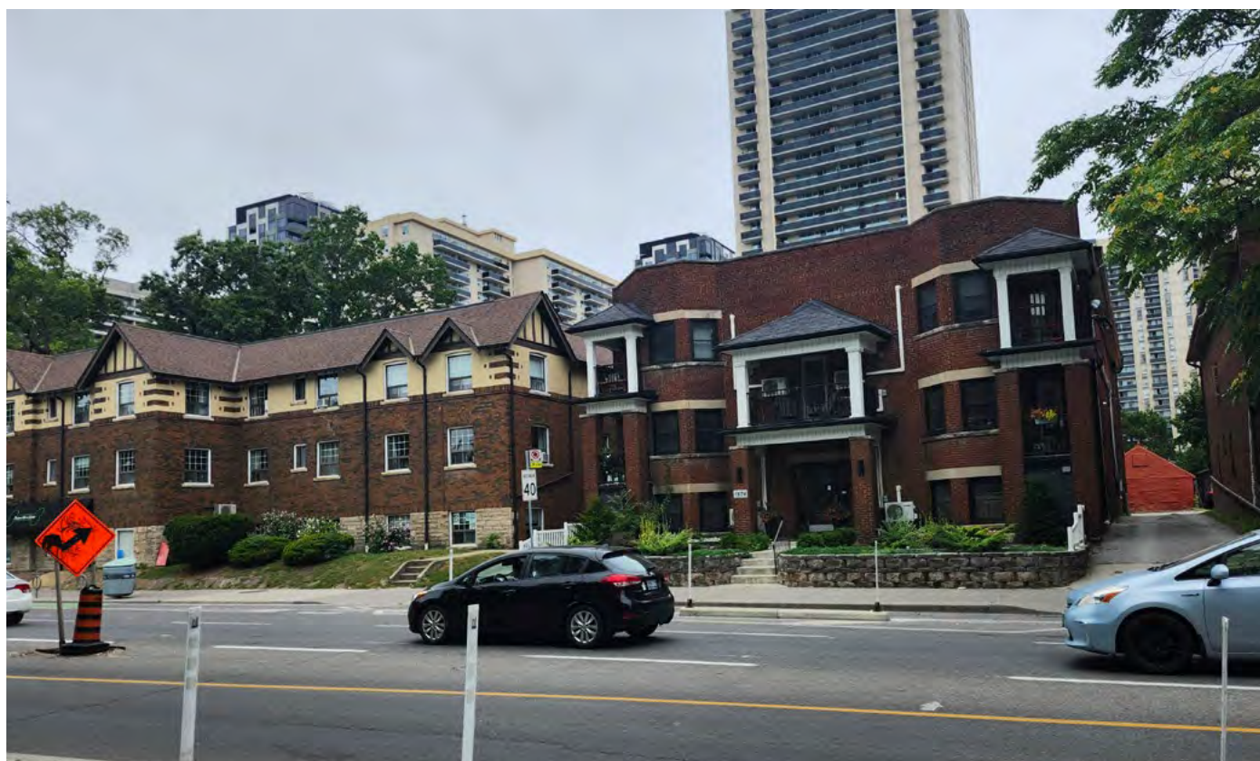
Low-scale walk-up apartment buildings within the High Park Frontage Character Area. (Credit: City of Toronto)
