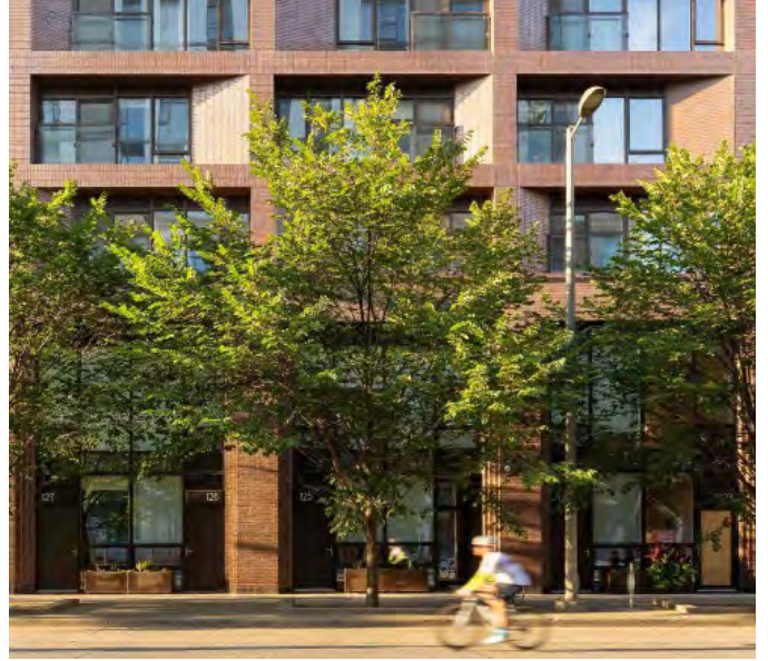
Maple House at Canary Landing exhibits high quality masonry material and detailing. Residential units at grade could accommodate home occupation uses with a live-work expression. (Credit: Artem Zavarzin)
