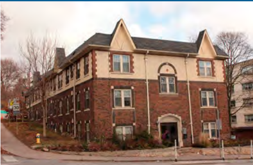
Showing principal (south) and west façades, looking northeast (Heritage Planning, 2023).
