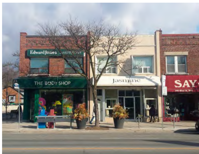
Main street commercial row buildings near the intersection of Willard Avenue Bloor Street West on the north side of the street. (Credit: City of Toronto)
