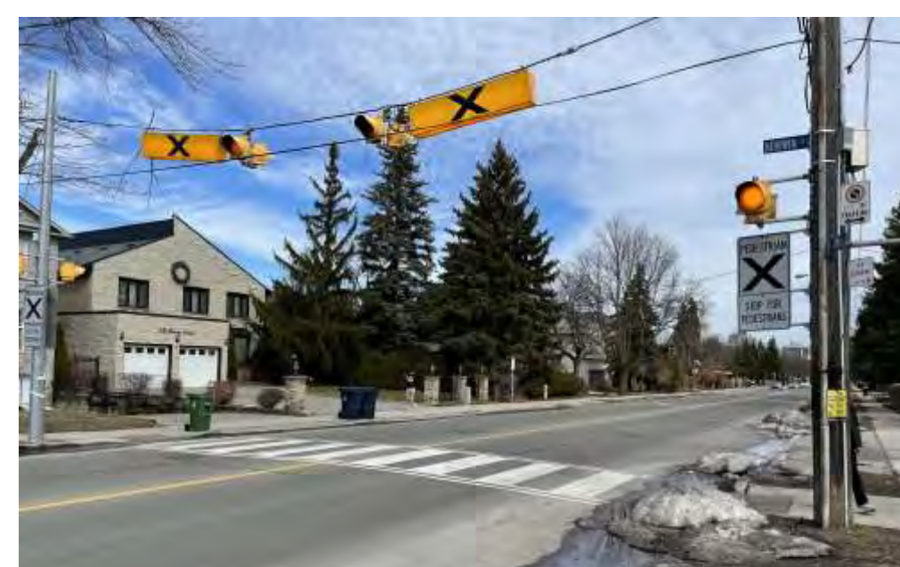
Drewry Lane facing east near R.J. Lang Public School
