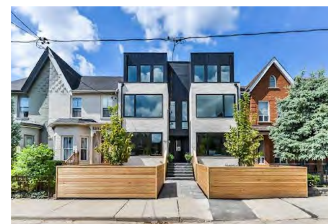
The South Annex, Toronto
