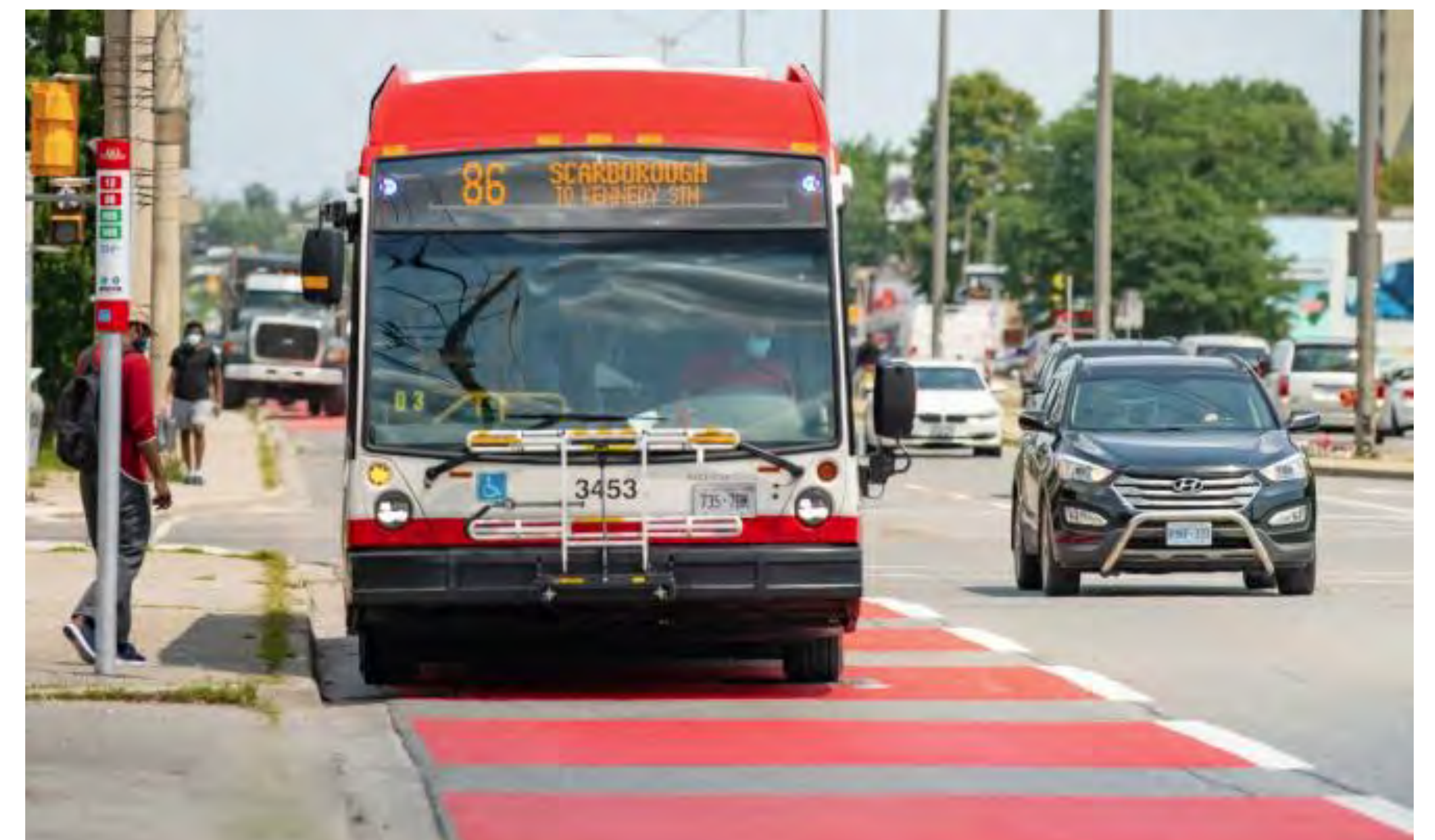
Priority Bus Lanes are one of the transit priority measures that can improve the reliability of transit service in Toronto.
