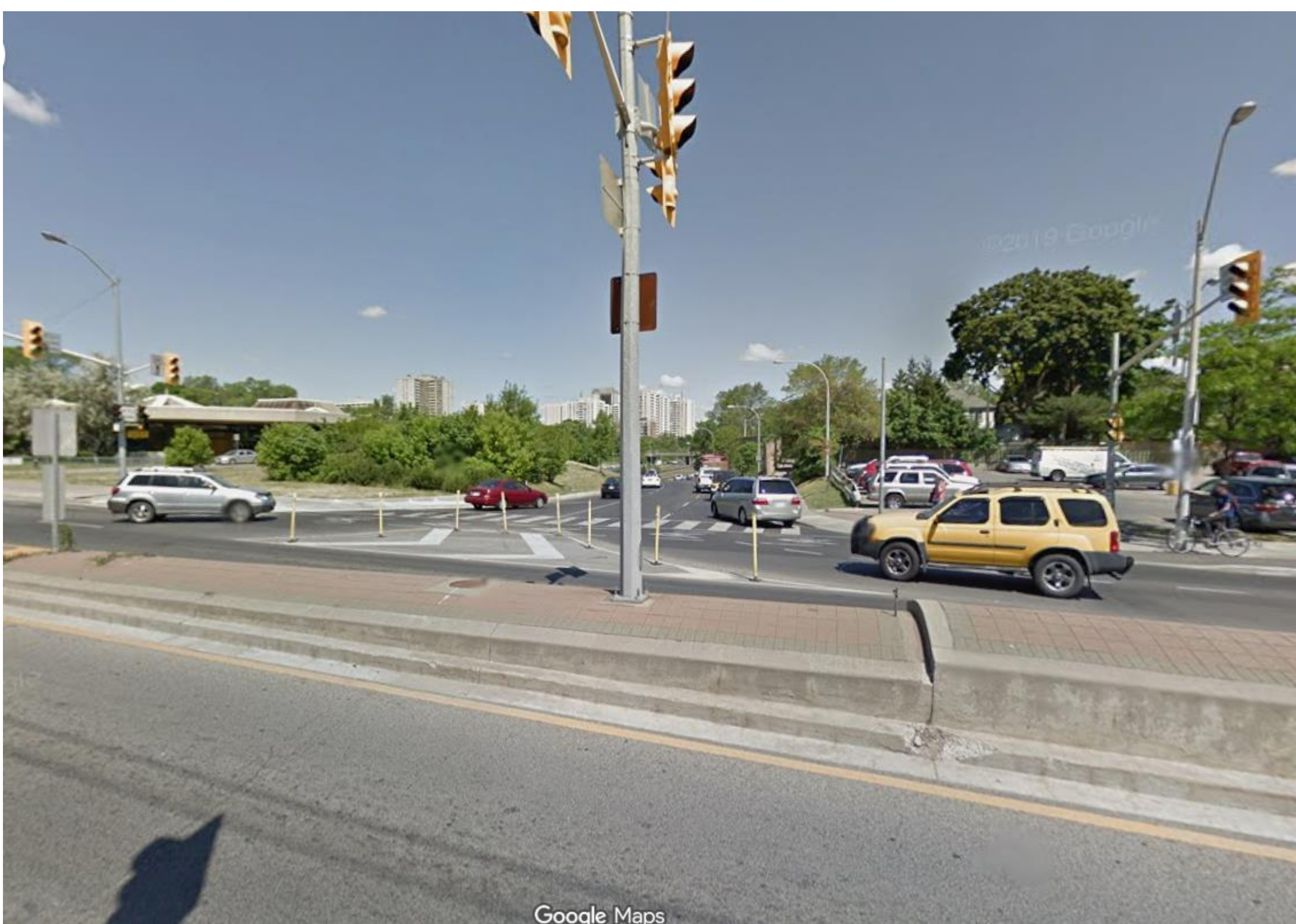
A view of the on-ramp in 2012 with three simultaneous turn lanes
