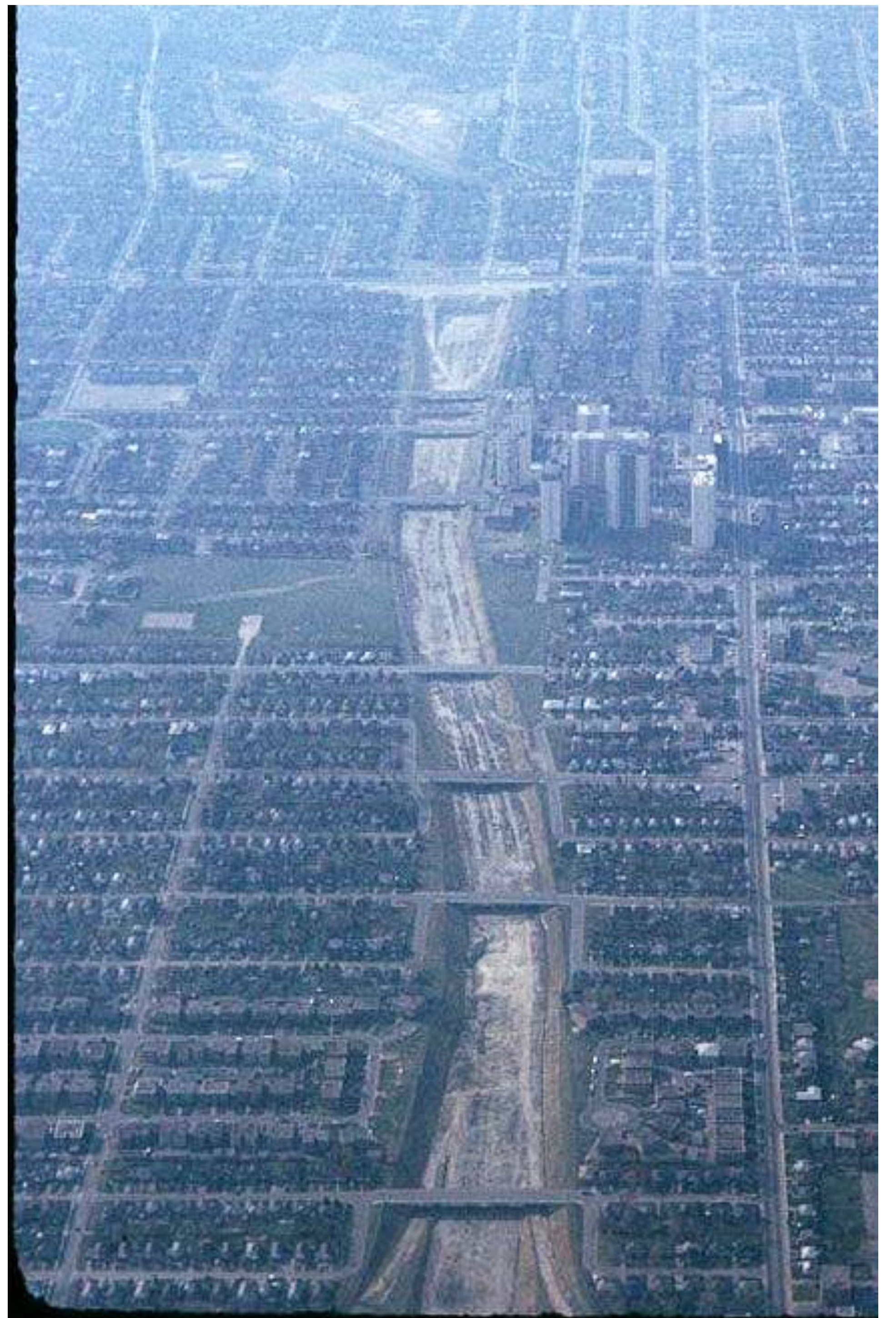
A view of Allen Road under construction between Lawrence Ave W and Eglinton Ave W in 1974.
