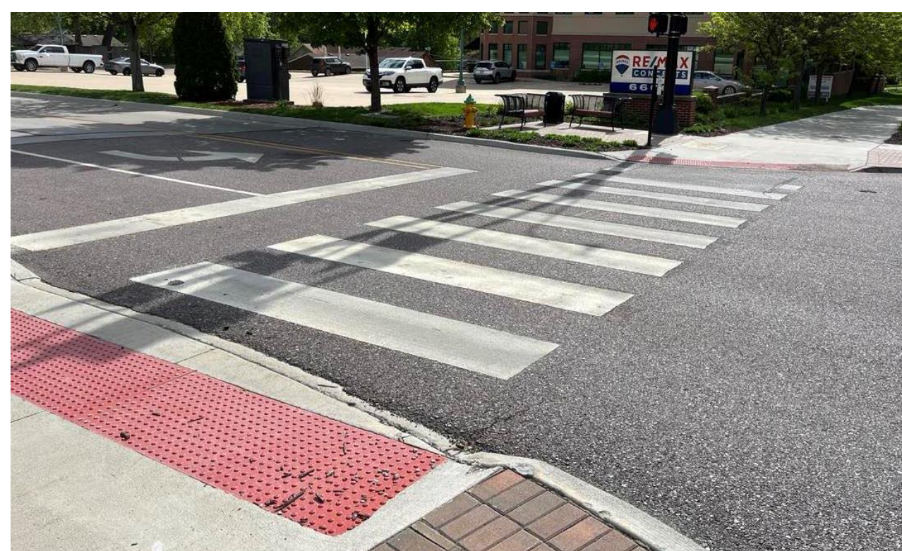
Addition of Missing Crosswalks
