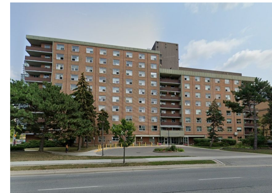
Mid Rise Building, Beecroft Road
