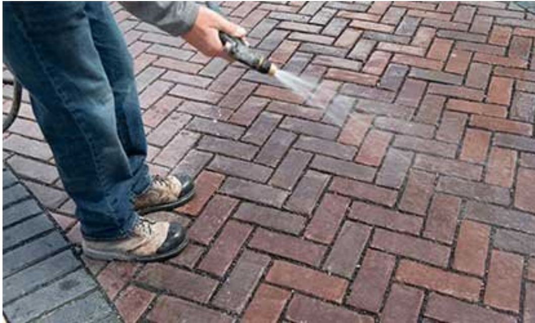
Demonstration of water filtering through permeable paver in roadway
