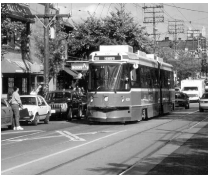
Move more people by giving streetcars and buses priority on City roads
