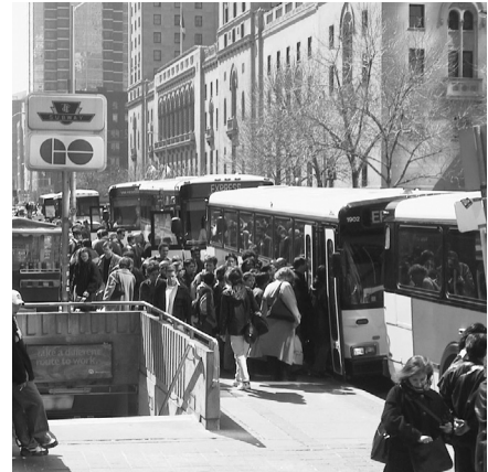
Union Station is a key transportation hub
