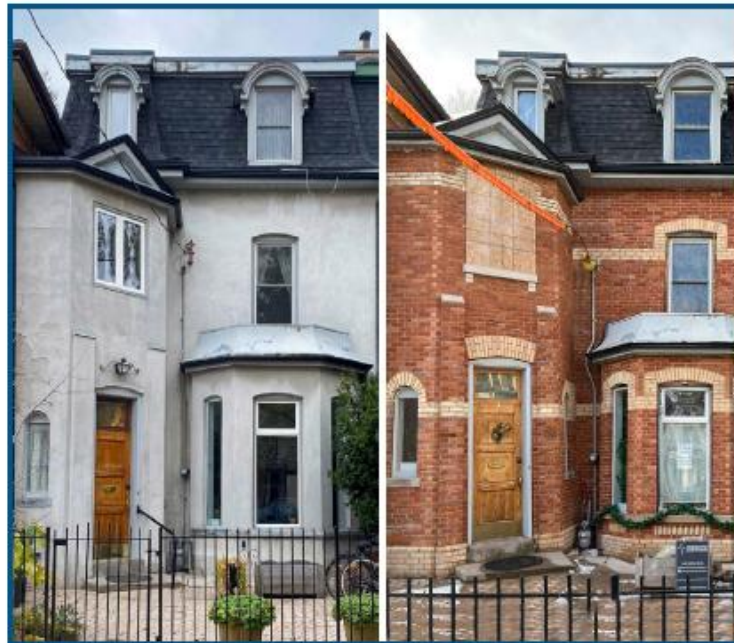
Heritage Grant Program | Funding support for masonry restoration was awarded to this property in the Cabbagetown Northwest Heritage Conservation District; Before conservation (left) and After conservation (right).
