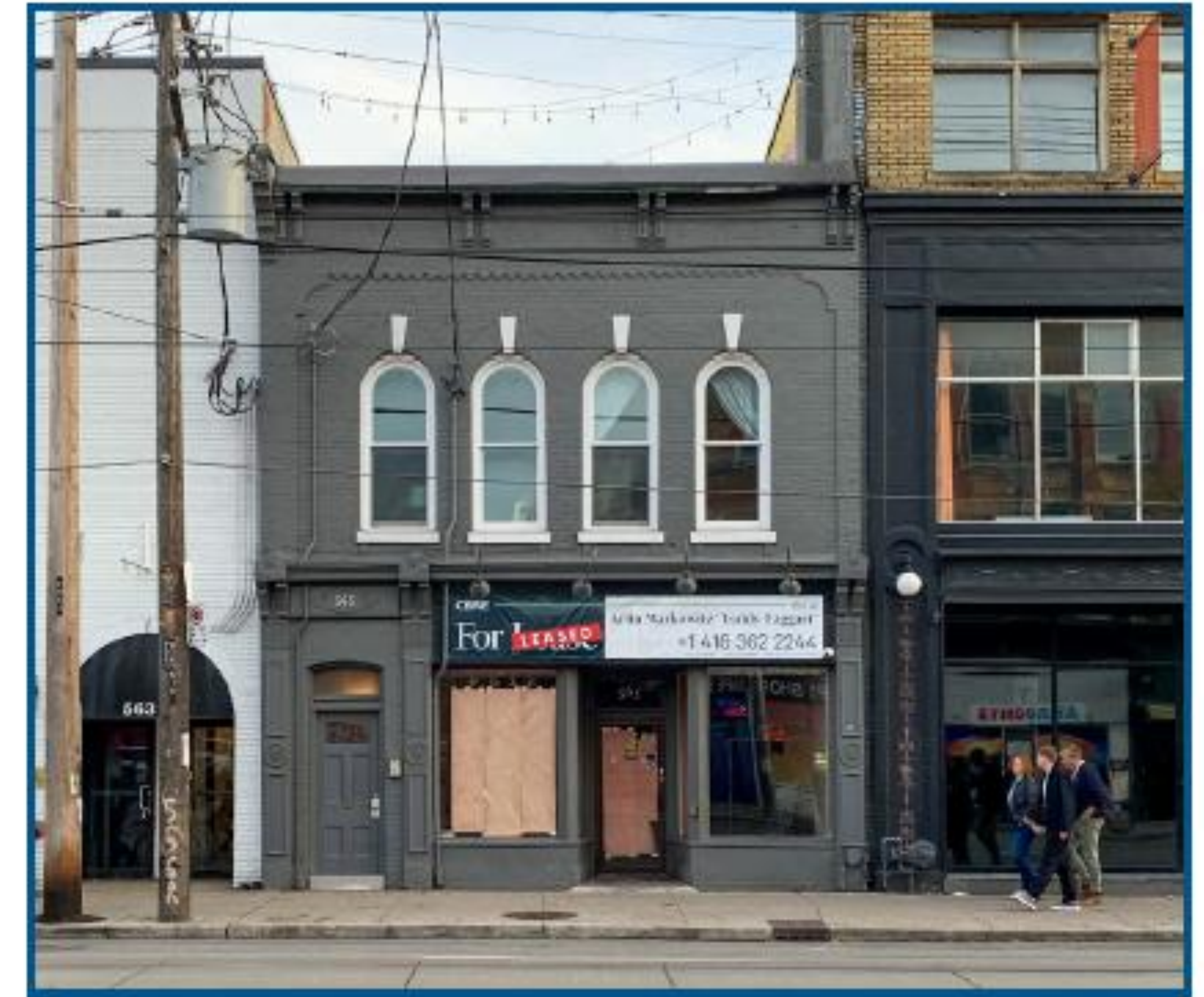
Heritage Property Tax Rebate Program | A commercial property in the Queen Street West Heritage Conservation District received funding support for window conservation.
