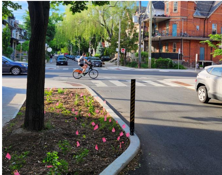
CURB EXTENSIONS Narrow local street intersections to slow vehicles down and reduce pedestrian crossing distance
