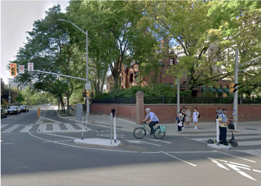
PROTECTED INTERSECTIONS Physically separate cyclists, pedestrians and vehicles to improve safety, visibility and comfort of all road users
