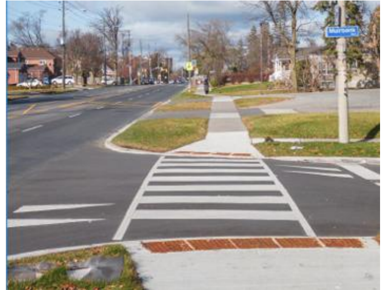
RAISED CROSSWALKS Elevate pedestrian crossings to slow vehicles down and improve pedestrian visibility and safety
