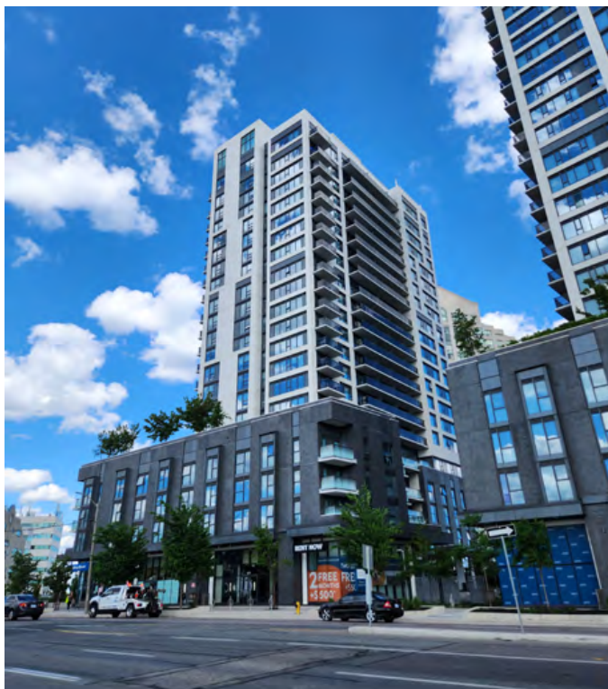
Precedent: 20 Samuel Wood shown as an example of a taller built form, prominent base building and tower portion perpendicular to the street and setback from the street. (Credit: City of Toronto)
