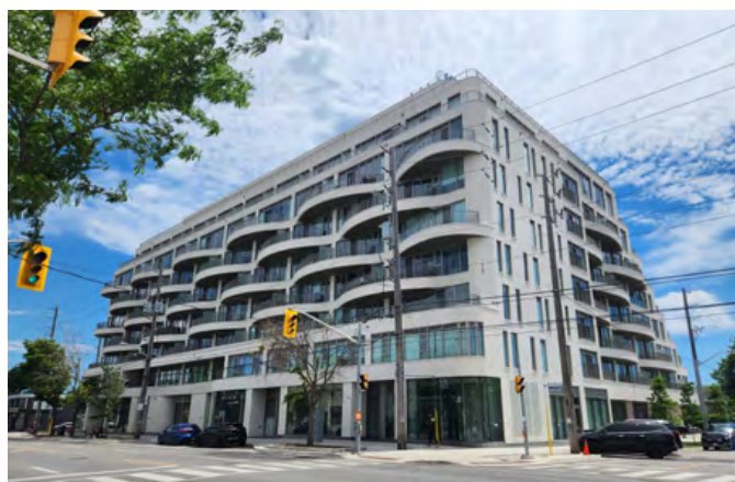
Precedent: 689 The Queensway (Reina Condos). Example of a 9-storey mid-rise building typology. (Credit: City of Toronto)
