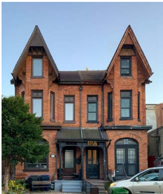
59 &amp; 61 Nassau Street (L-R)
