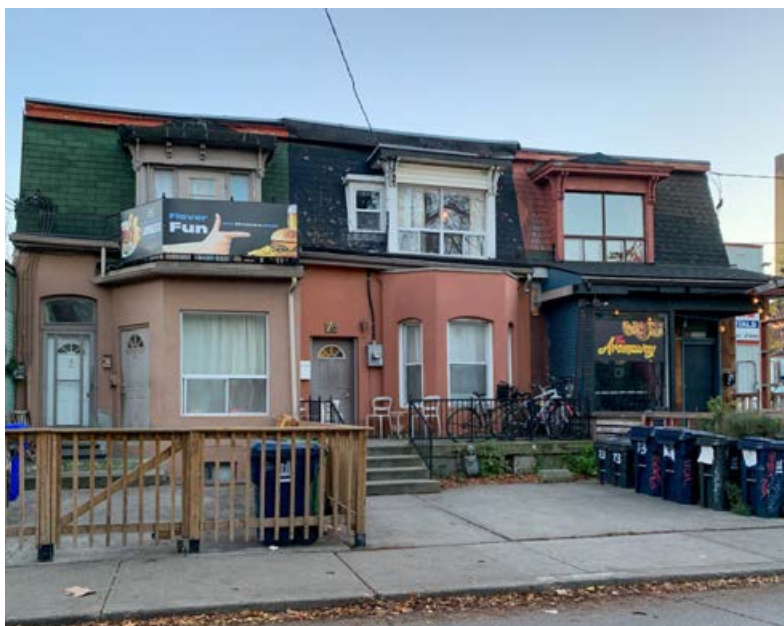
71, 73, &amp; 75 Nassau Street (L-R)
