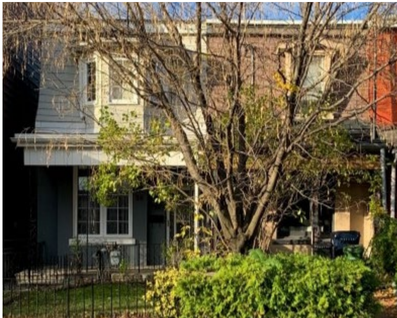
36 & 38 Lippincott Street (L-R)
