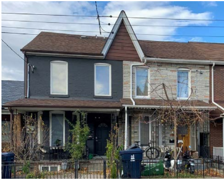
16 & 18 Lippincott Street (L-R)
