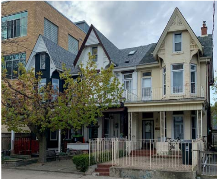
29, 31, &amp; 33 Nassau Street (L-R)
