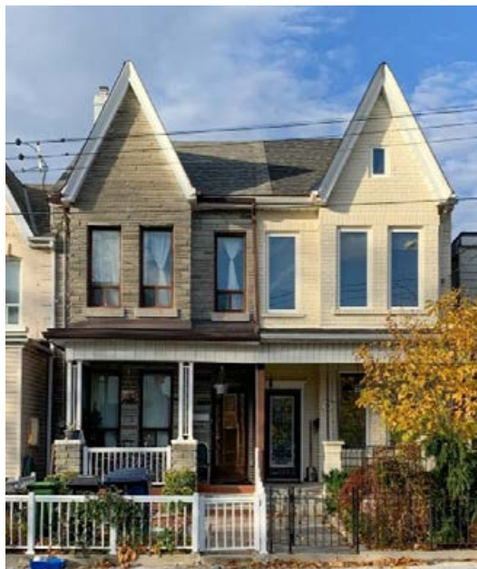
32 & 34 Lippincott Street (L-R)
