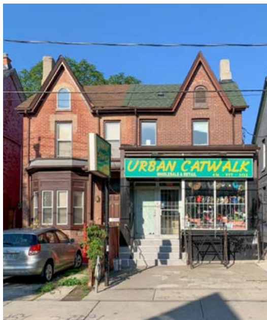
8 &amp; 10 Kensington Avenue (L-R)
