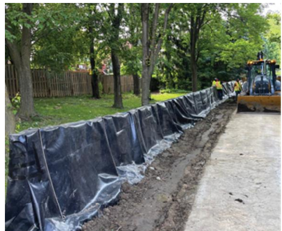
Temporary flood mitigation using modular flood barriers
