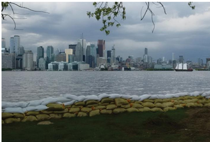
Temporary flood mitigation using sandbags
