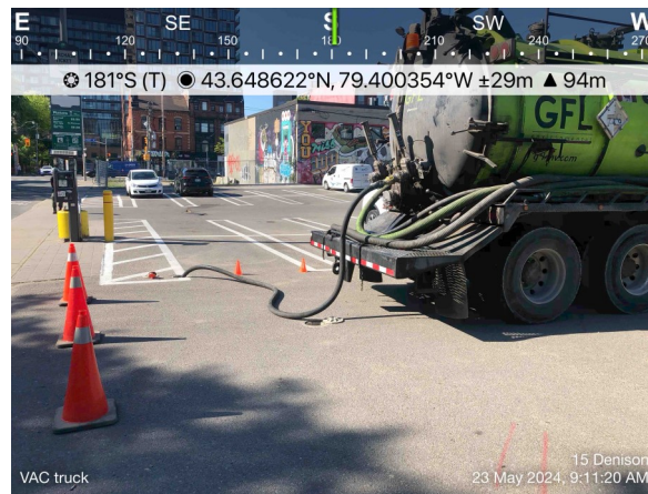
Photo 2: View of extraction set up. Photograph taken facing south.
