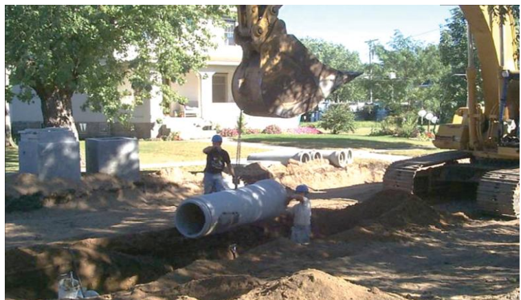
Photo showing installation of new sewer pipe
