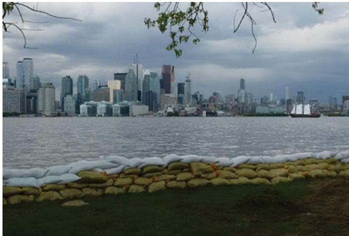
Temporary flood mitigation using sandbags
