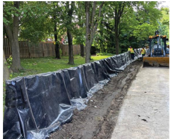
Temporary flood mitigation using modular flood barriers
