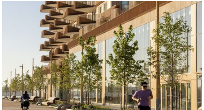
Figure 35. Double height glazing and warm colours contribute to an attractive facade. Vertical facade elements create a series of segments along the length of the building contributing to a comfortable pedestrian scale. (East Bayfront Community Centre)
