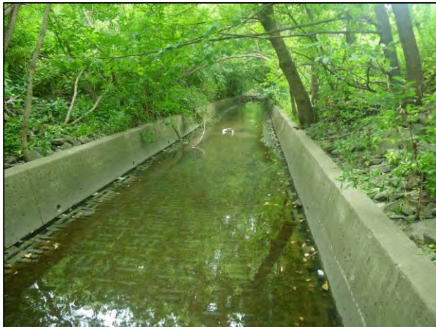
Facing upstream at channel lined with concrete blocks and bordered by near-vertical concrete walls and steep rip rap slopes
