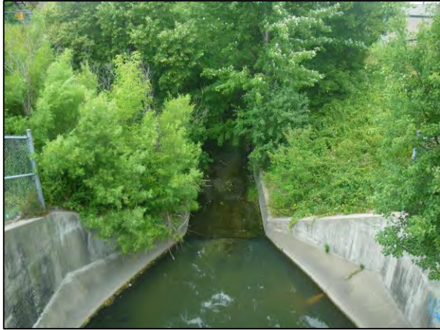
Upstream facing upstream (northwest) from top of culvert crossing of Ashtonbee and Birchmount Roads
