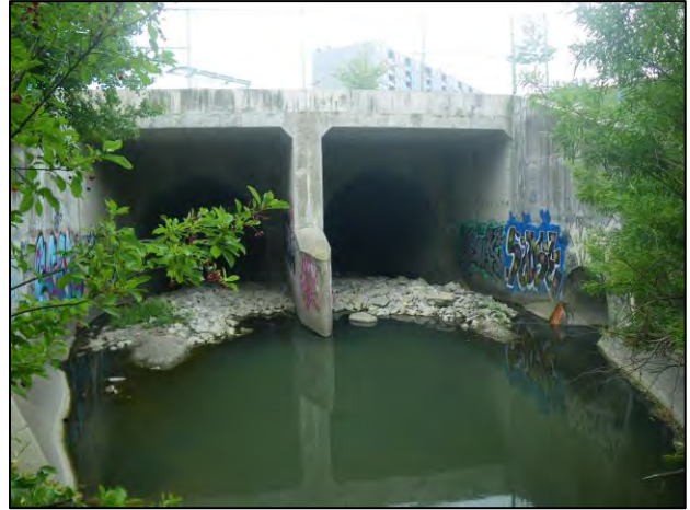
Upstream (north) end of twin CSP culvert under Ashtonbee and Birchmount Roads
