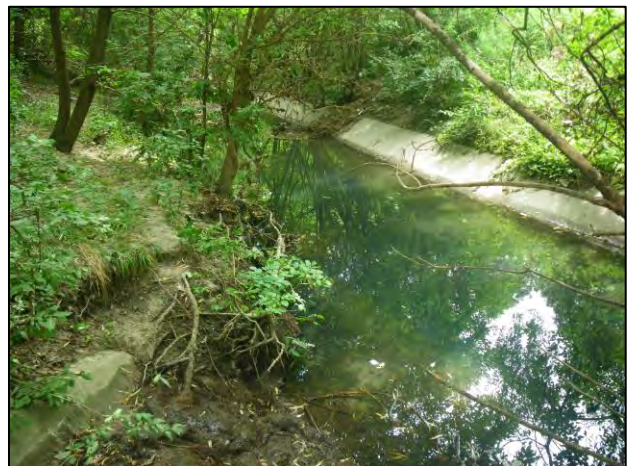
Downstream channel facing downstream (southeast). Note that channel is more trapezoidal here compared with upstream but lined concrete banks and steep riparian slopes
