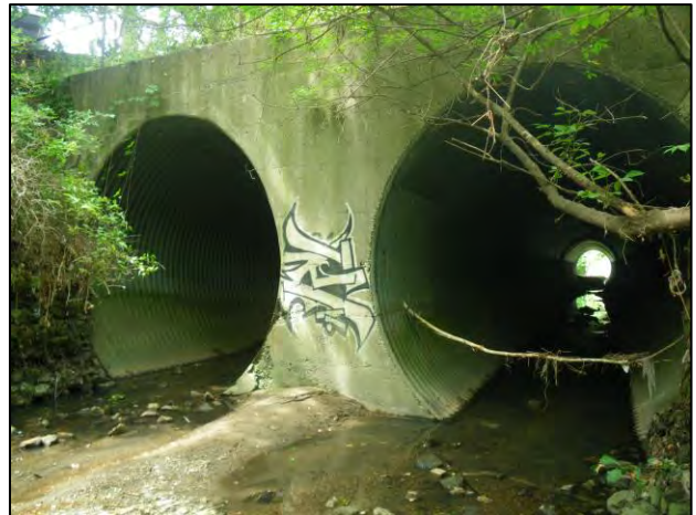
Downstream facing upstream (northwest) at downstream ends of CSP culverts under Ashtonbee and Birchmount Roads
