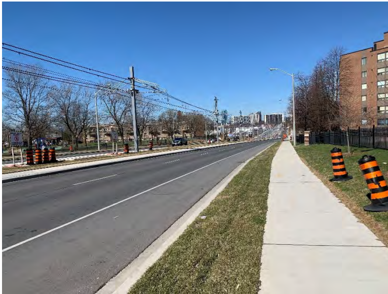
Plate 1: Eglinton Avenue East, looking west from west of Victoria Park Avenue. Note the L.R.T. under construction in the middle of the road (A.S.I. 2022).
