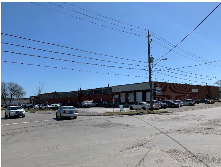
Plate 8: Typical low rise industrial building within the study area, looking southeast from intersection of Manville Road and Sherry Road (A.S.I. 2022).
