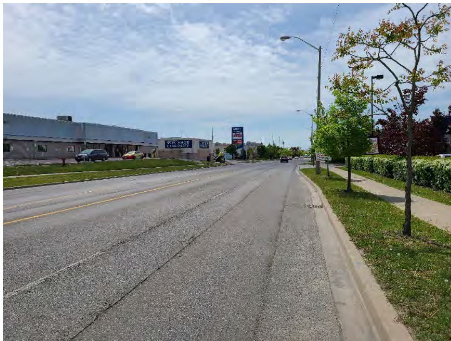
Photo 6: View to the southeast of the Lebovic Avenue roadway from 2 Lebovic Avenue.
