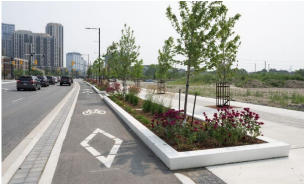
Figure 7-10: Raised Planting Zone and the Cycle Track (Dundas Street)
