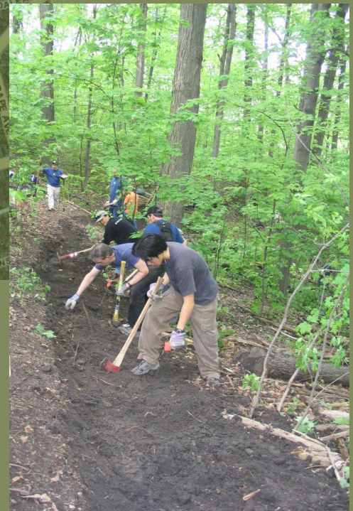
New Trail Construction
