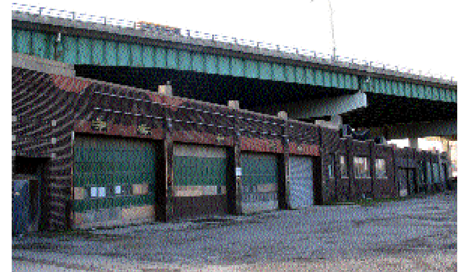
View of existing one-storey warehouse building, looking southwest
