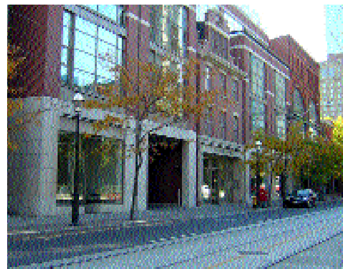
Service access integrated with retail frontage – King Street East, Toronto
