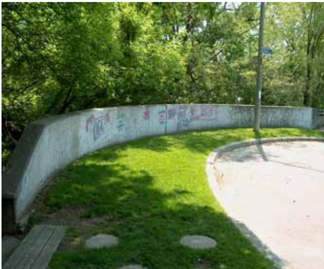
Entrance to greenbelt
