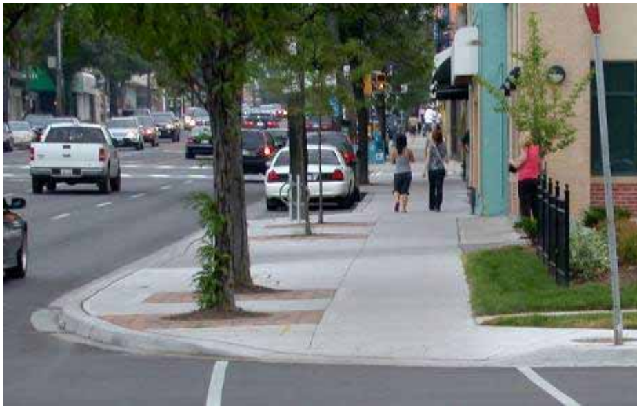
Parking bump-outs along Avenue Road.
