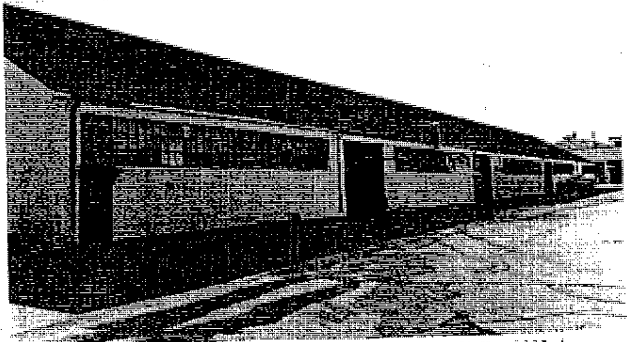
37 Storage Building #42, west side elevation. (DND, 1990.)
