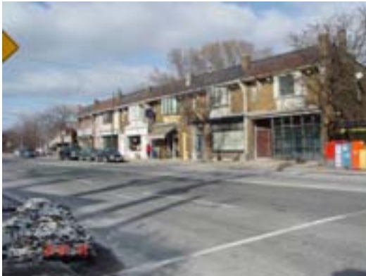
Existing prewar mainstreet buildings east of Birchcliff Avenue.
