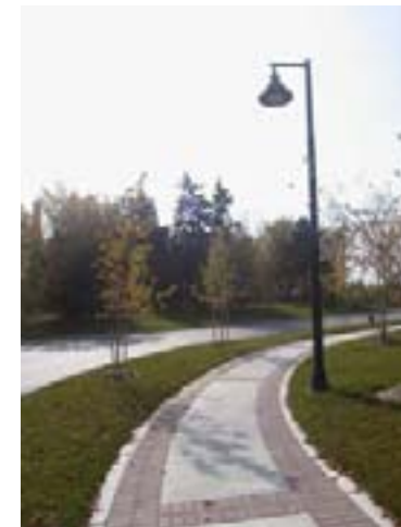
Pedestrian pathway with decorative lighting & paving material.
