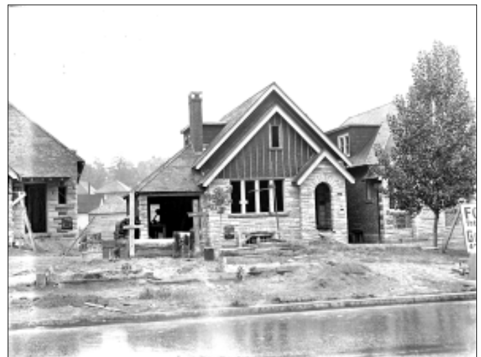
Construction on the Kingsway, June 17, 1936, SC 266, Item 40448
