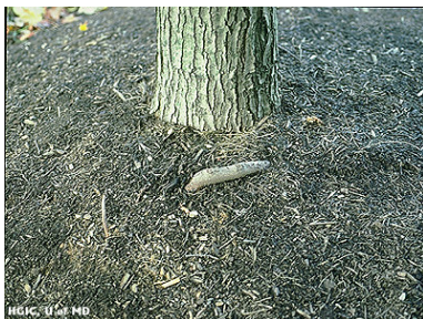
Lack of butt flare at the base indicates the presence of girdling roots
