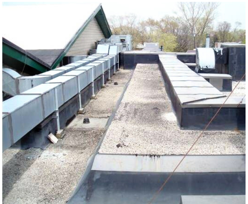
Before Eco-Roof installation
