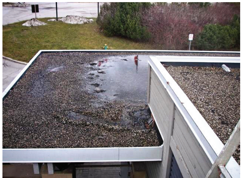
Before Eco-Roof installation
