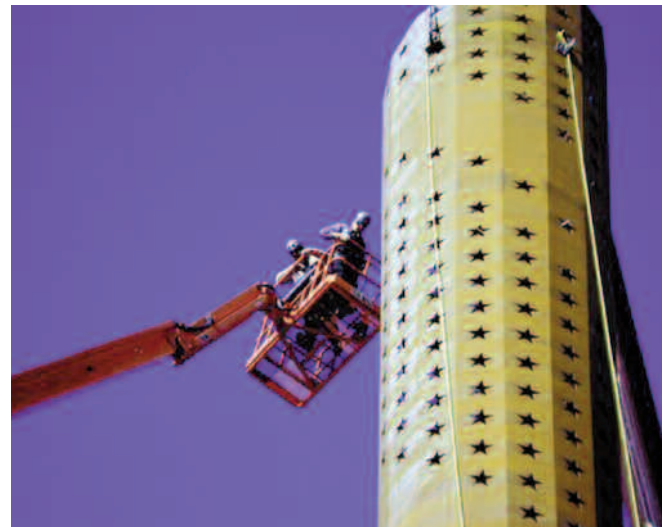
Public art under construction
